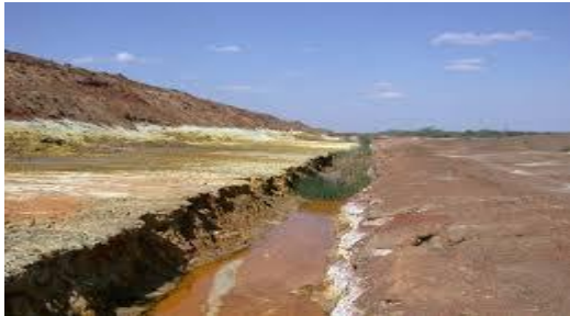
(b) Acid mine drainage from tailings dump in BCL mine
