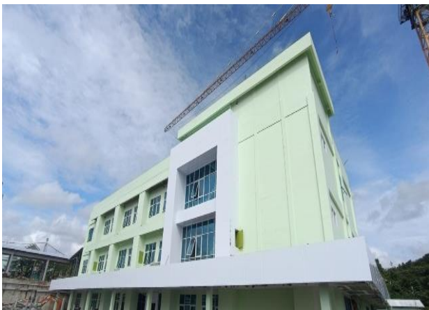
Fig 6. View of building 5, Aji Muhammad Parikesit General Hospital
