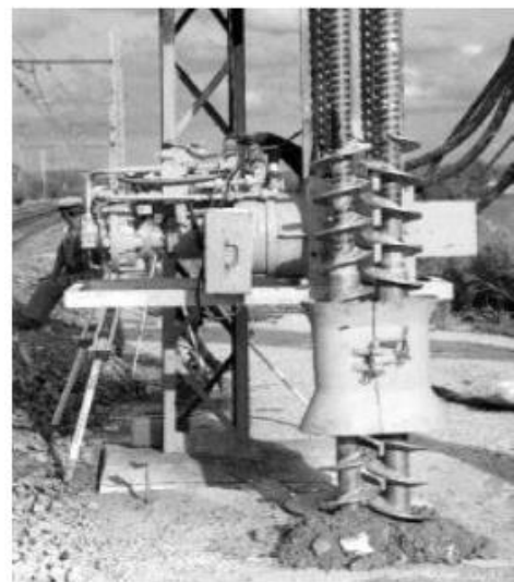
Fig. 8. Installation of lime column in the field using Colmix method (Larsson, 2002)
