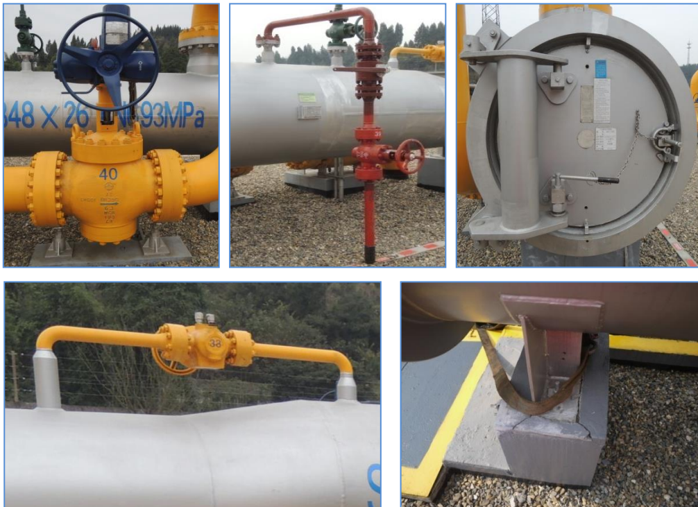
Fig. 3. Components of the pig launcher
