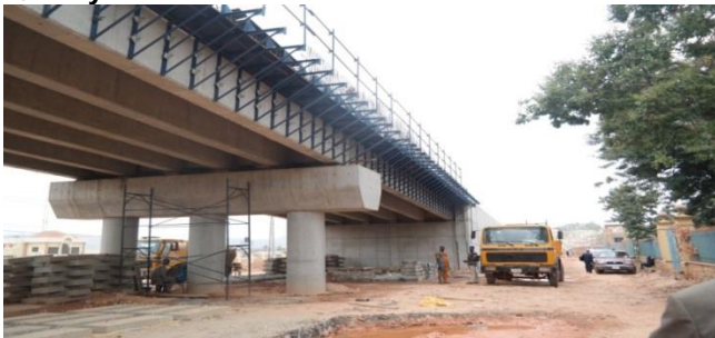
Plate 3: Construction of Fly-over at Fajuyi Ado-Ekiti
