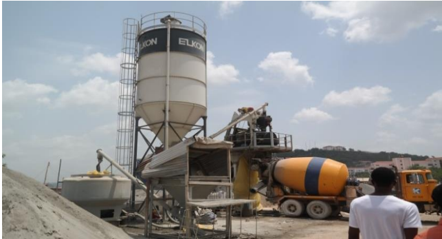
Plate 2: Mixing of Concrete for Adequate Quality
