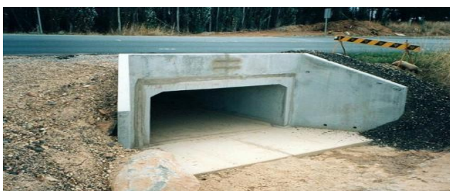
Fig 1: A simple culvert
