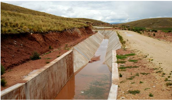
Fig. 2 A simple channel transition
