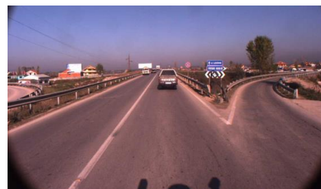
Figure 4 Road entrance in Fushkrujë, SH2,x 436,1460,y 28.39, km 16 + 655 m
