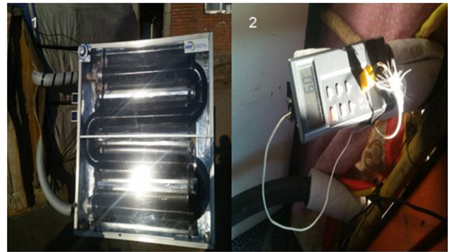
Fig. 4. 1.actual air heating system 2.checking collector output temperature
