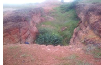
Plate 4: Abandoned pit by Bisichi-Jenta showing relative displacement in Rahei-Larwin
